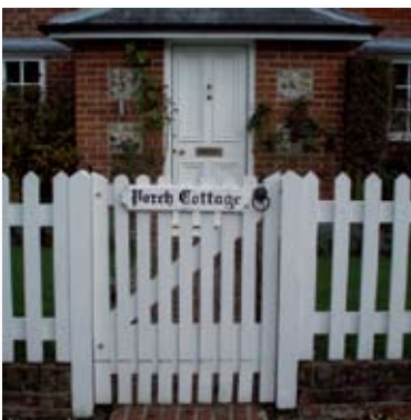
Picket fence and gate, Porch Cottage
