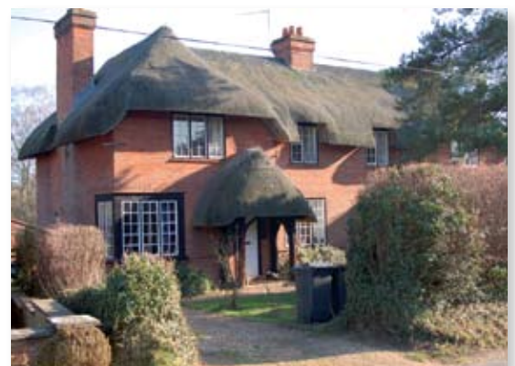
Nos 1 and 2 Lavender Cottages
