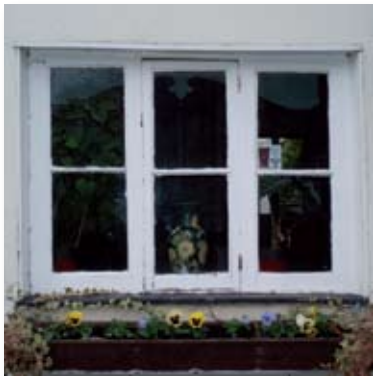
Hampshire casement window, Crook and Shears Public House
