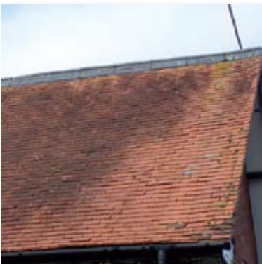
Clay tile roof, Old School
