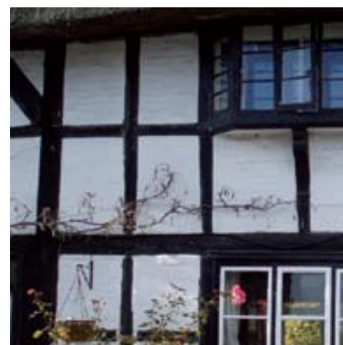
Timber framing, Queen Anne Cottages
