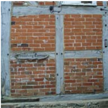
Timber framing, Boundary Cottage
