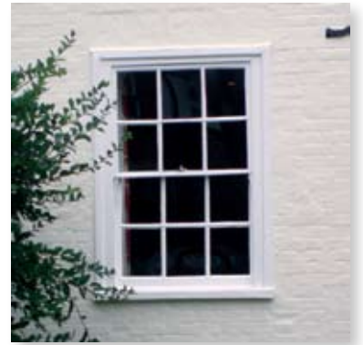
Sash window, Hollies
