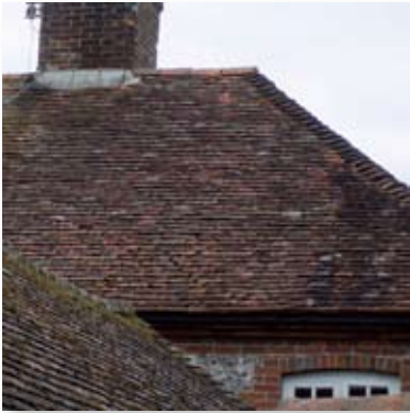
Clay tile roofing, Parsonage Farm
