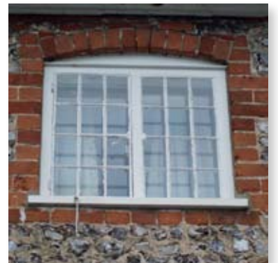
Metal casement window, Maltings
