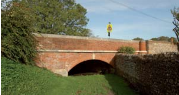
Bridge over the River Swift
