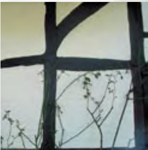
Timber framing with infill panels of brick
