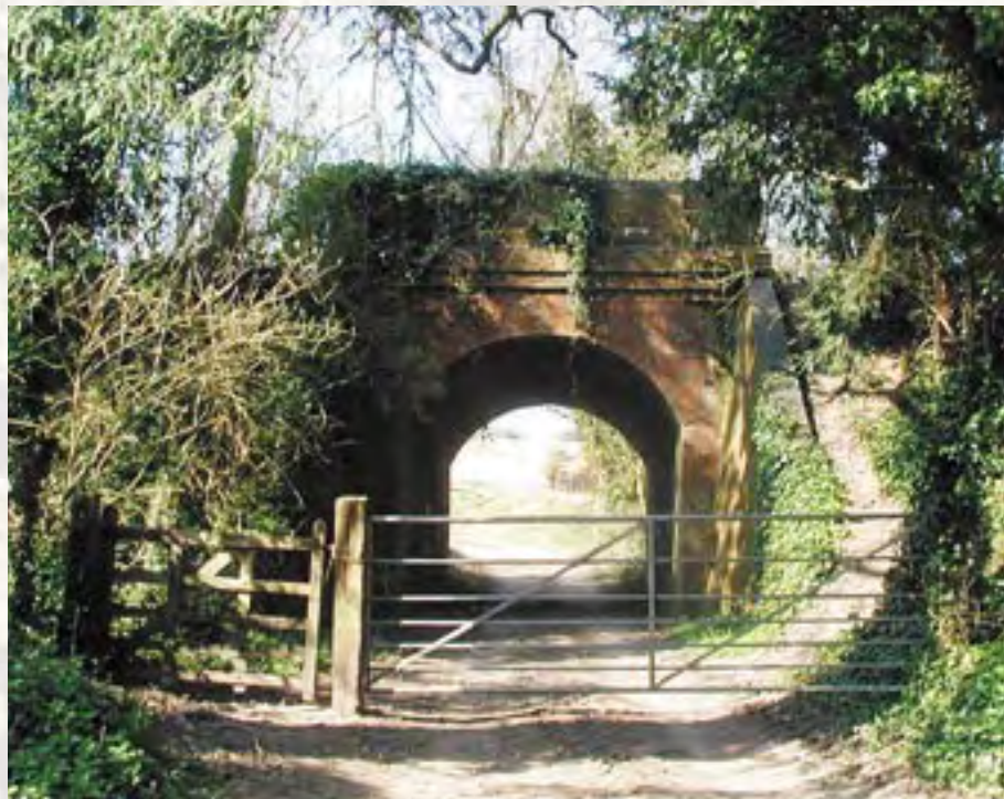
Bridge over former railway line
