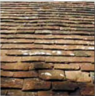
Clay tiles, Rectory, Church Street
