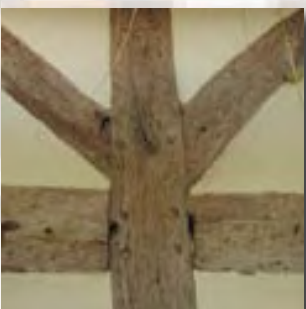
Timber framing, with infill panels of plaster, Mole Hall, Church Street
