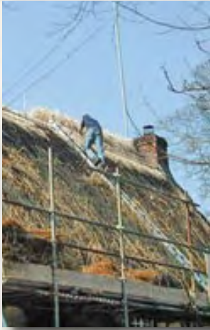
Thatching in progress
