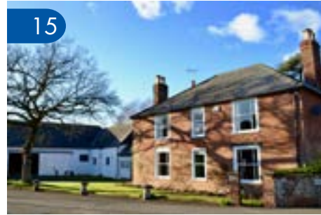
Church Farm house, Village St.
