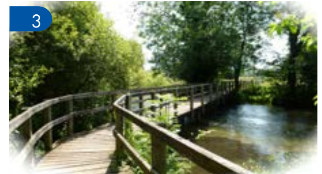
3 Chilbolton Cow Common from Wherwell entrance
