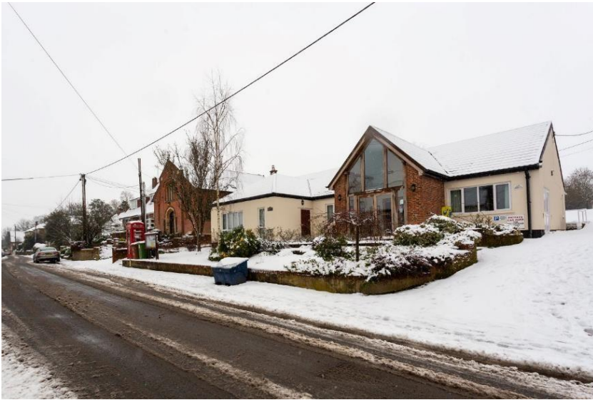
Upper Clatford Village Hall
