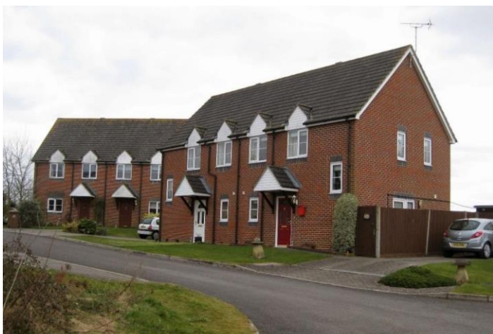
Village housing at Alexander Close
