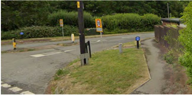
Current shared cycle paths are narrow and poorly surfaced
