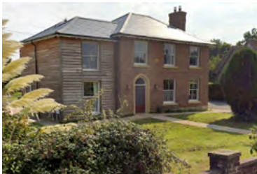
Here, a new dwelling was constructed in a traditional form, with what appears to be an example of a contemporary contrasting extension. In fact this constructed at the same time.
