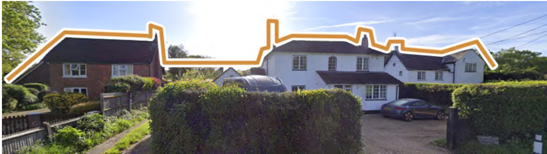
Example of the varied building heights in a street adding interest to the street scene. Note that the changes in height are proportionate and one building does not dominate another or cause problems with overlooking and loss of privacy through careful placement of windows.
