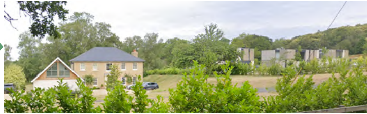
New buildings of a mix of significantly contrasting styles, without any continuity or reference on a site should be avoided
