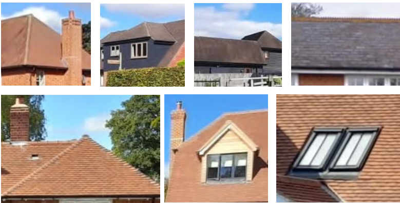
PA.II - ROOF MATERIALS AND FORM - Simple roof forms - hipped and half hipped predominate
