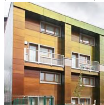
Ernley Close, Manchester (Source: 2e Architects)
