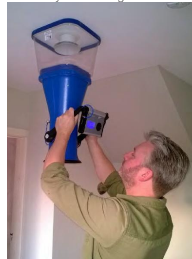
Flow rate measurement: image of MVHR system being commissioned (Source: Fourwalls)
