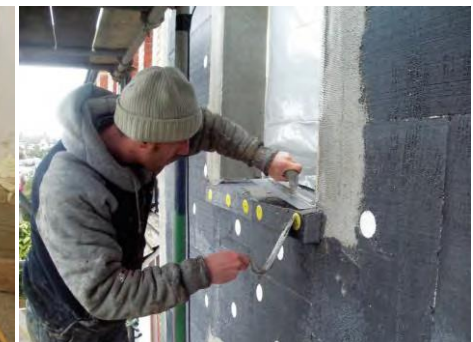
Window install in EnerPHit retrofit (Source: Passivhouseplus)
