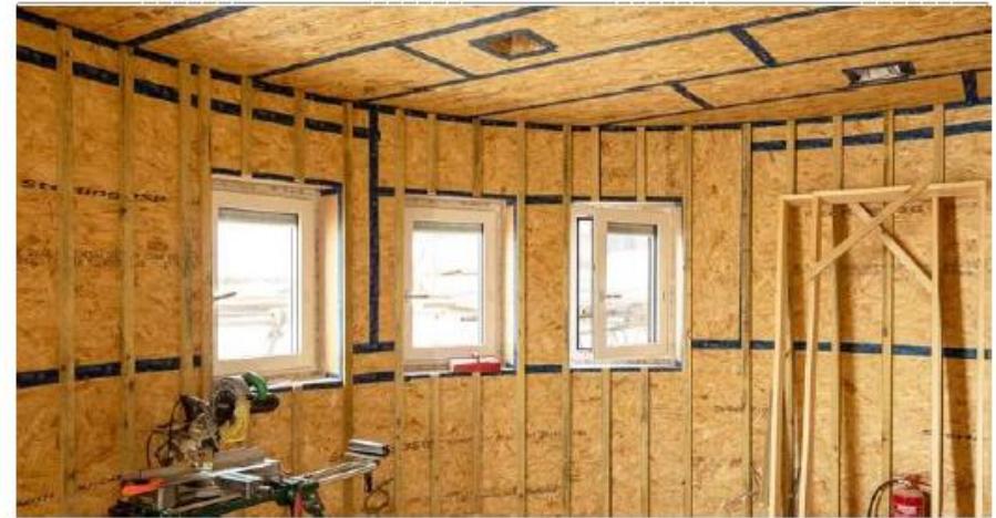
A good airtightness strategy forms the basis of an airtight building. This is an excellent example of taped OSB, with a dedicated service cavity on internal walls. The service cavity means most wires and pipes will not breach the airtight OSB layer.
