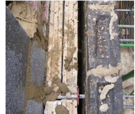
Left: an example of good Expanded Polystyrene insulation installation. Right: An example of poorly installed partial cavity installation, loosely fitting, and cement dropped atop and inside cavity (Source: Etude)
