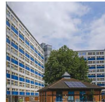
Wilmcote House, Plymouth (Source: ECD Architects)
