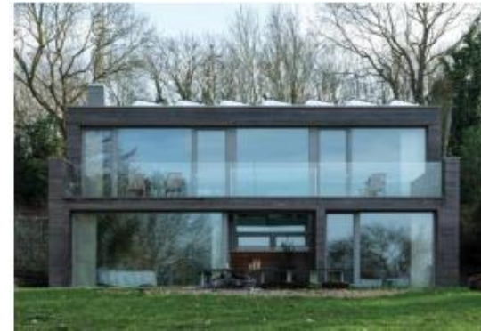
Lark Rise, Chiltern Hills. Passivhaus Plus certified. (© Bere:architects)
