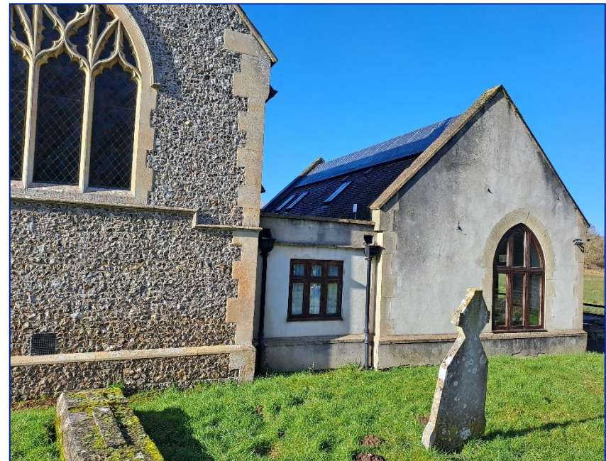
Principal and prominent pitches should be kept free from Solar Panels, to minimise visual impact, or placed on extensions or buildings of less significance
