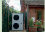
Air Source Heat Pump situated in the Garden behind screening
