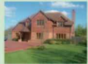
Installation 14 Kw Heat Pump with Domestic Hot Water
