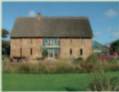
Barn conversion Heat Pump installation featured in Grand Designs
