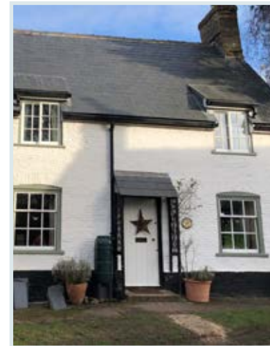
Figure 60: Examples of water butts used for rainwater harvesting in Reach, Cambridgeshire.
