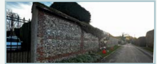
Flint stone wall with red brick detailing
