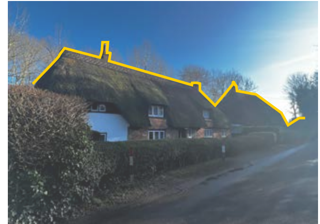
Figure 17: Traditional Hampshire style thatched roofs with wrapover ridges and red brick chimney stack in East Cholderton, the low-lying nature of the roofscape allows for mature vegetation to create a natural backdrop.
