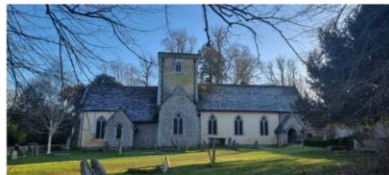
Church of St Mary Grade II* Listed
