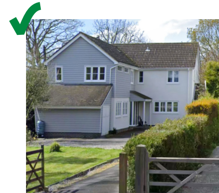
Here, a 1970s dwelling has been extended and refurbished with high quality materials.
