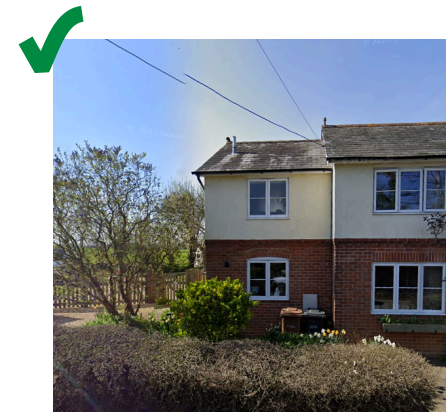
Extension too close to boundary with insufficient space for landscaping.
