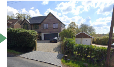
Replacement 2 storey contemporary dwelling. Frontage hedge and trees have been removed
