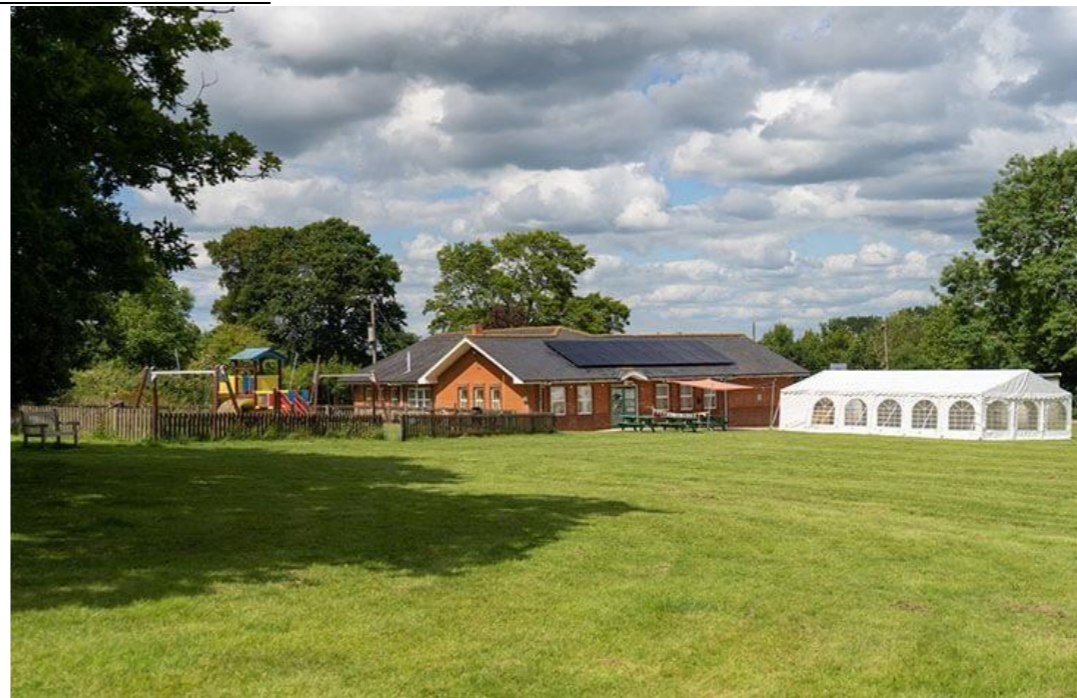
Figure 40. Awbridge Village Hall 5
