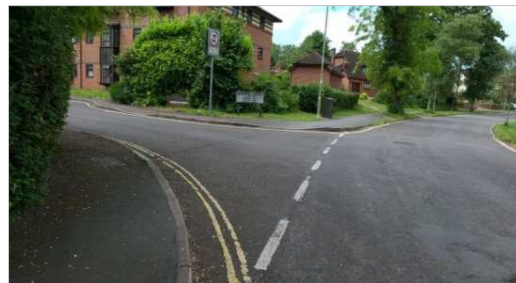
WR1.7.1 – Bishops Way and Junction Road junction
