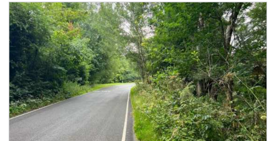
100.1.11 – End of Leyton Path and Watery Lane
