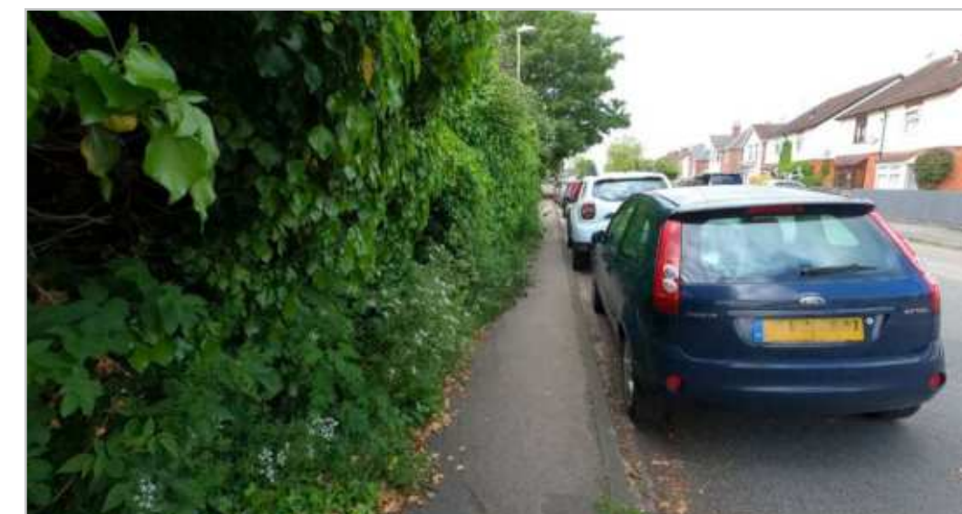
WR1.3.3 – Vigo Road pavement
