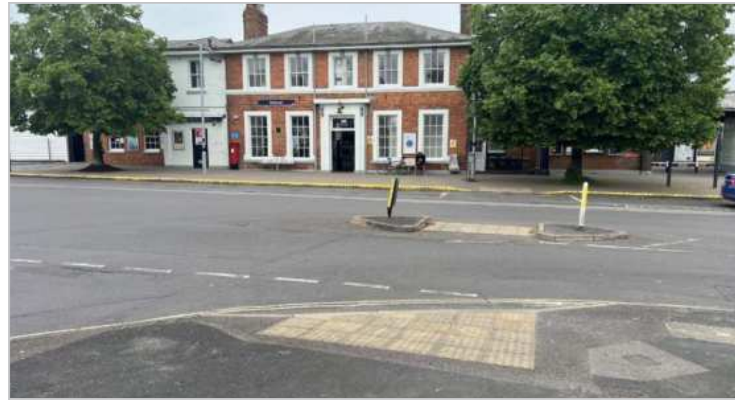
200.1.7 – Andover railway station entrance
