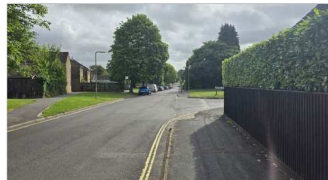
230.1.1 – London Road Access Road conditions
