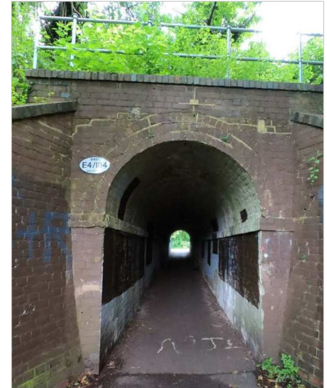
WR1.1.9 – Railway underpass north of Enham Arch retail park
