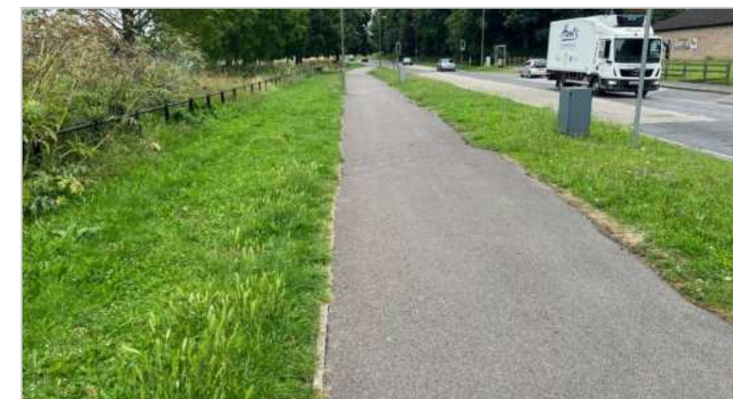
220.1.3 – Shared use facility on Smannell Road
