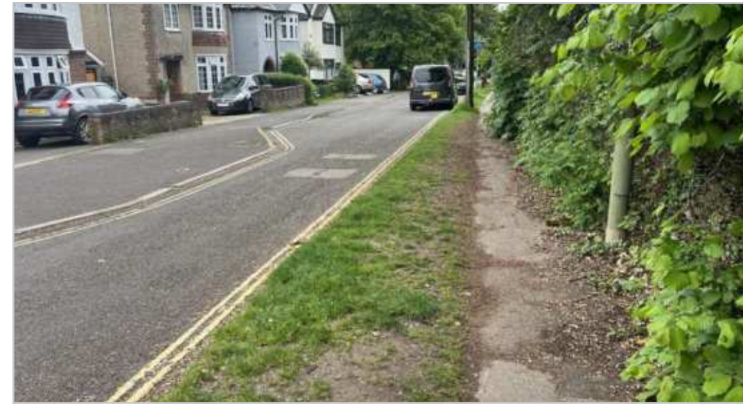
200.1.10 – Junction Road footway
