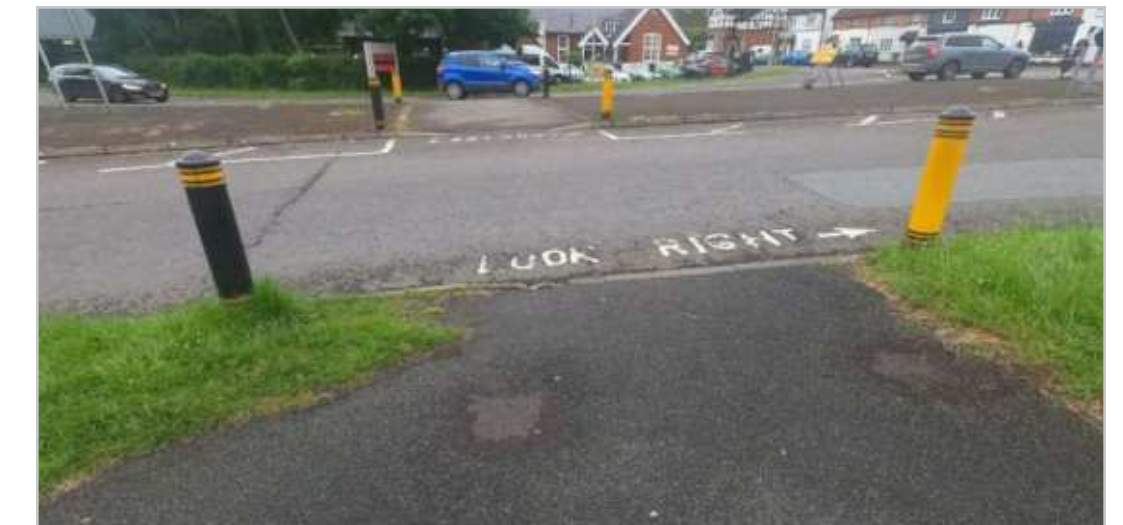
W22.1.10b – Crossing Point over Winton Hill arm of A30 roundabout
