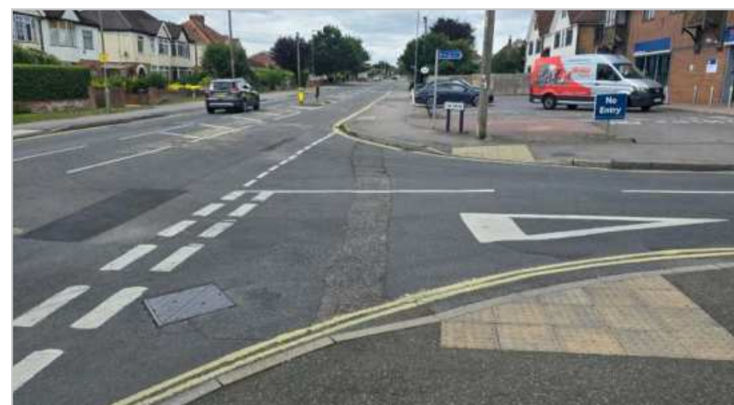
200.1.3 – Weyhill Road junction with The Drive
