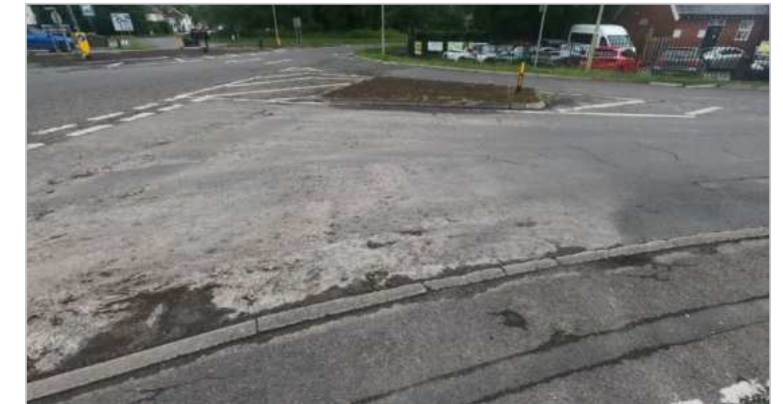
W22.1.10a – A3057 arm of the A30 roundabout
