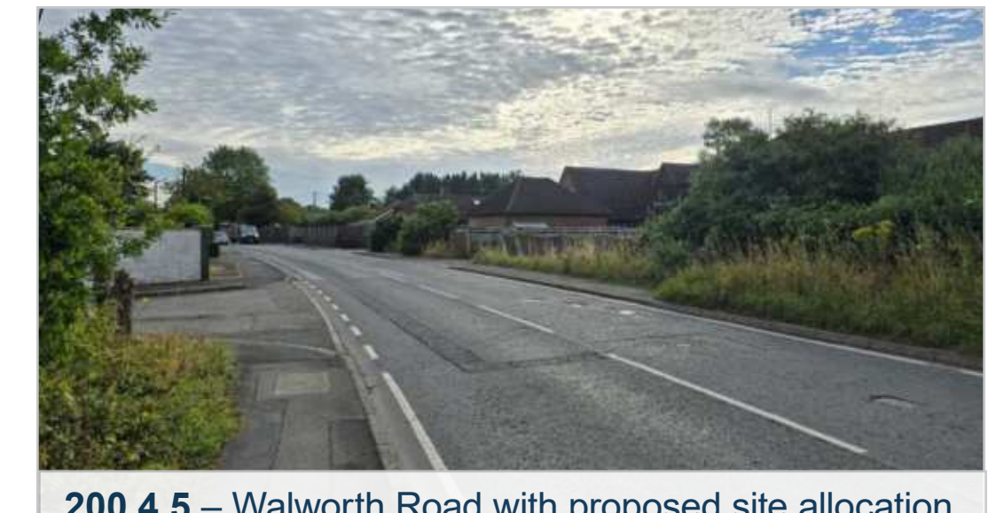
200.4.5 – Walworth Road with proposed site allocation to the right of the photo
