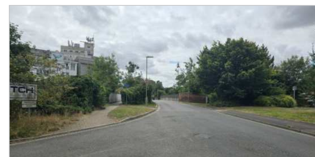
200.1.5 – Railway Bridge at the junction of Watson Acre and Millway Road
