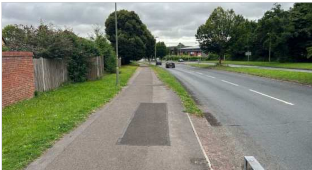
110.1.6 – Newbury Road near railway bridge
