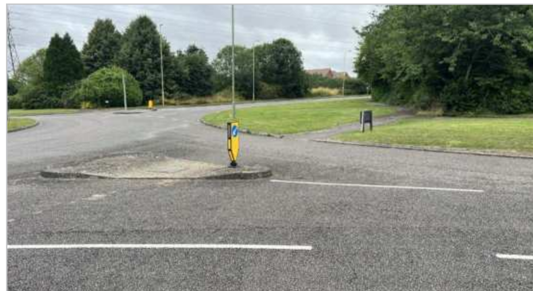
100.1.2 – Saxon Way/Goch Way roundabout
