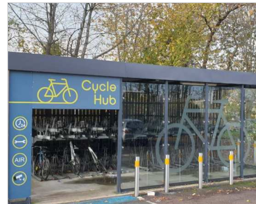
An example of cycle hub parking facilities – Winchester Train Station
