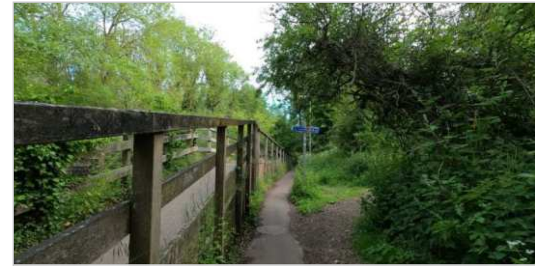
WR1.1.7a – Footpath conditions behind Enham Arch retail park
