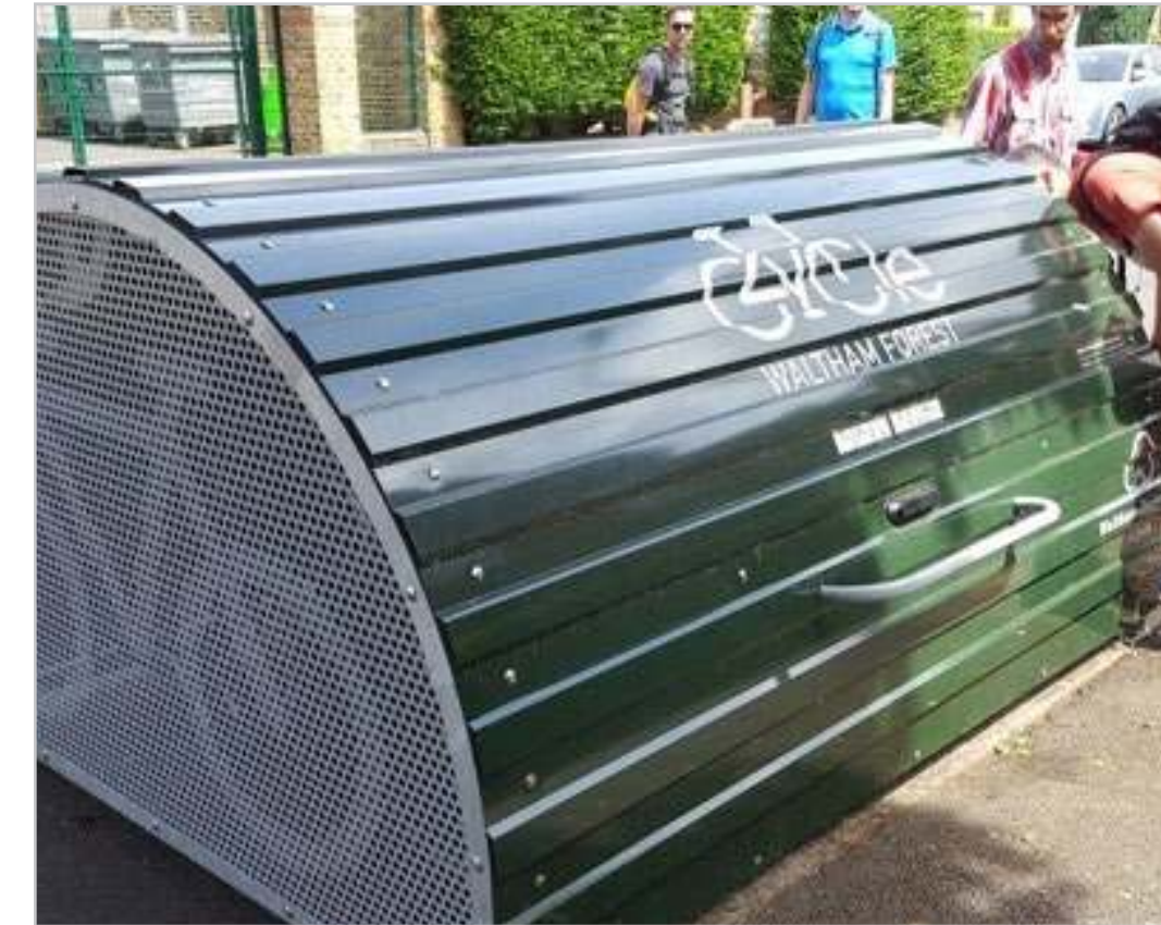
An example of on street lockable cycle 'hangar' style parking facilities – Waltham Forest, London
