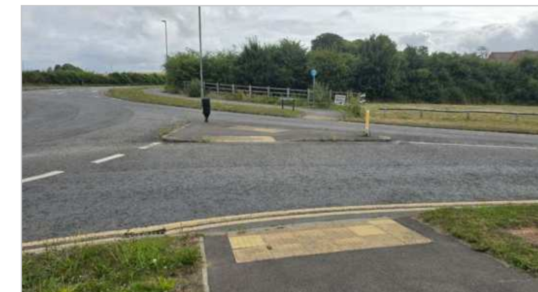
230.1.3 – Picket Twenty roundabout
