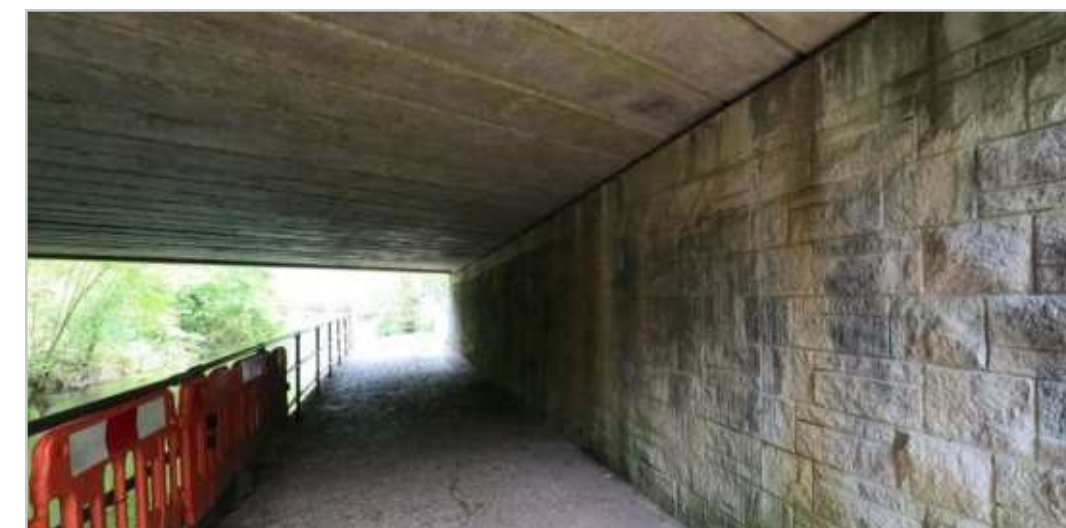
WR1.1.8 – Pedestrian underpass beneath Northern Avenue
