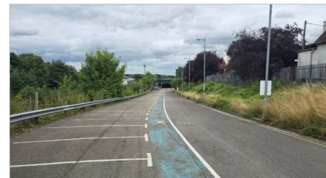
200.1.6 – Route through the railway station car park
