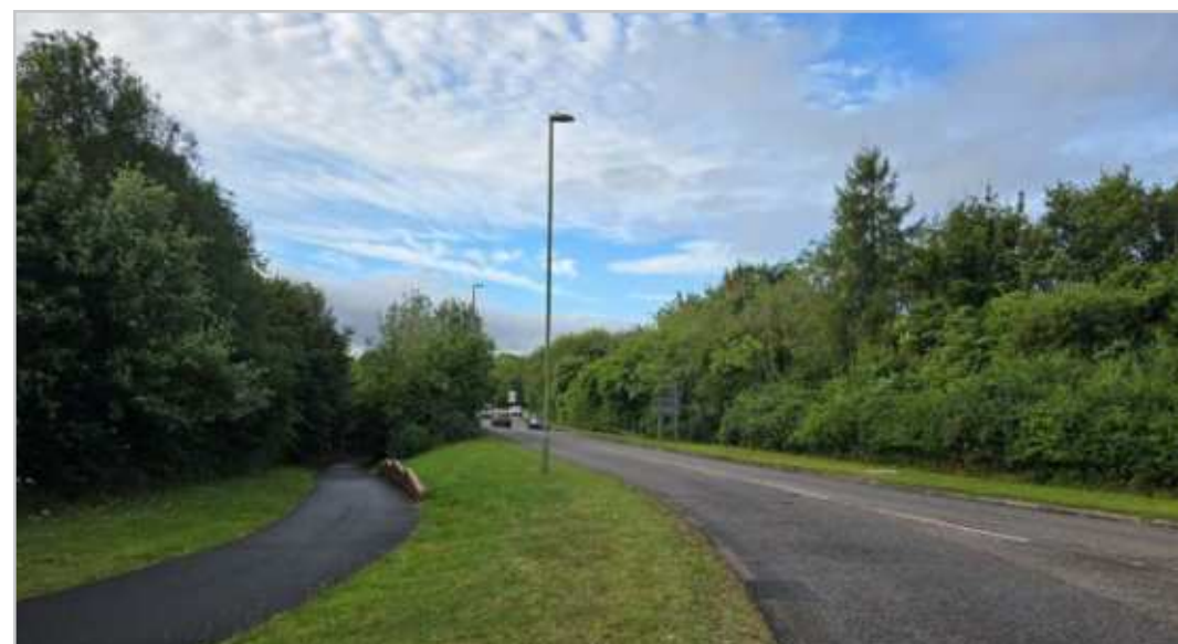
100.1.3 – Goch Way and Parallel Footway
