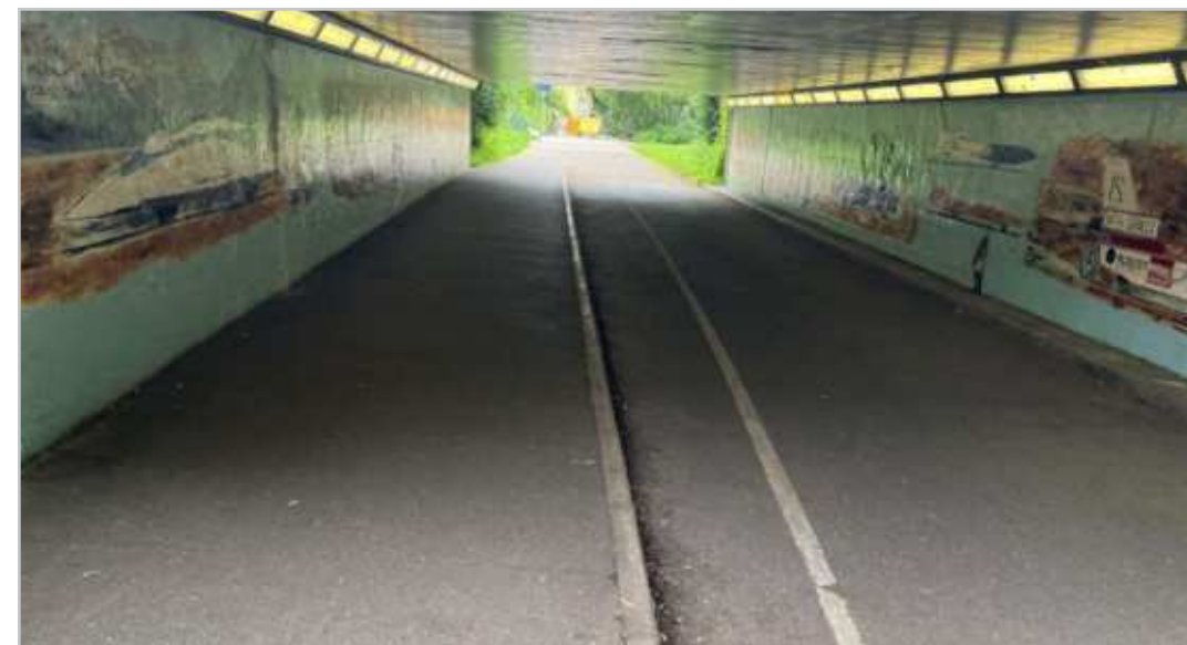
200.1.11 – Underpass beneath Western Avenue
