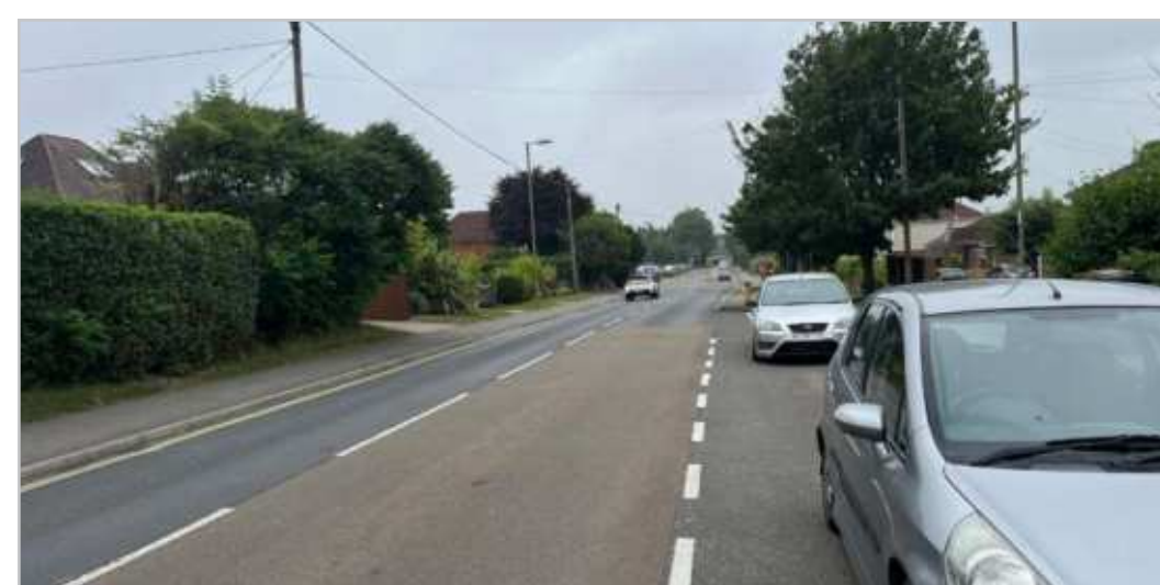
200.1.2 – Weyhill Road conditions east of Weyhill roundabout
