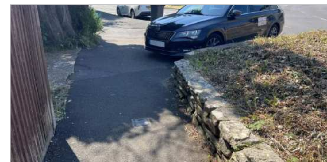
WR1.7.4b – Planting area considered for redevelopment as part of the Station Approach scheme
