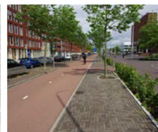
Coloured Asphalt Cycleway and Clay Paver Footway / Monolithic poured material with clay pavers.
