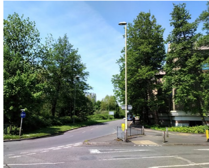
Southern entrance to site
