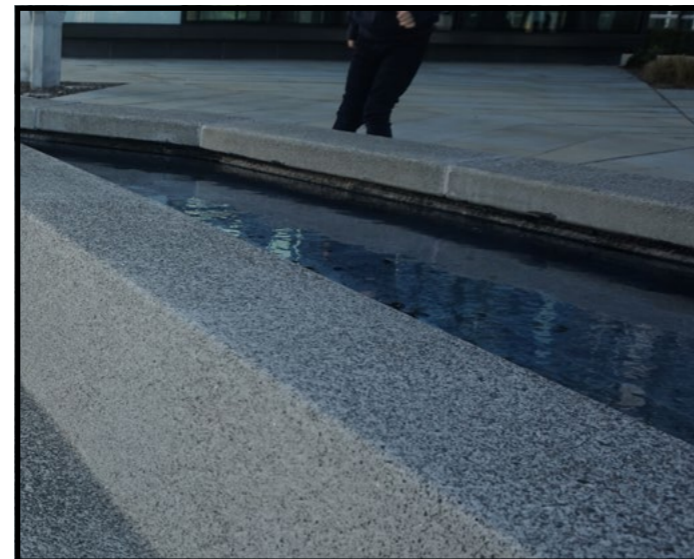
2) Water feature - Rill within raised concrete wall
