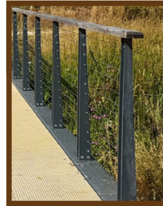
Balustrade to walkway
