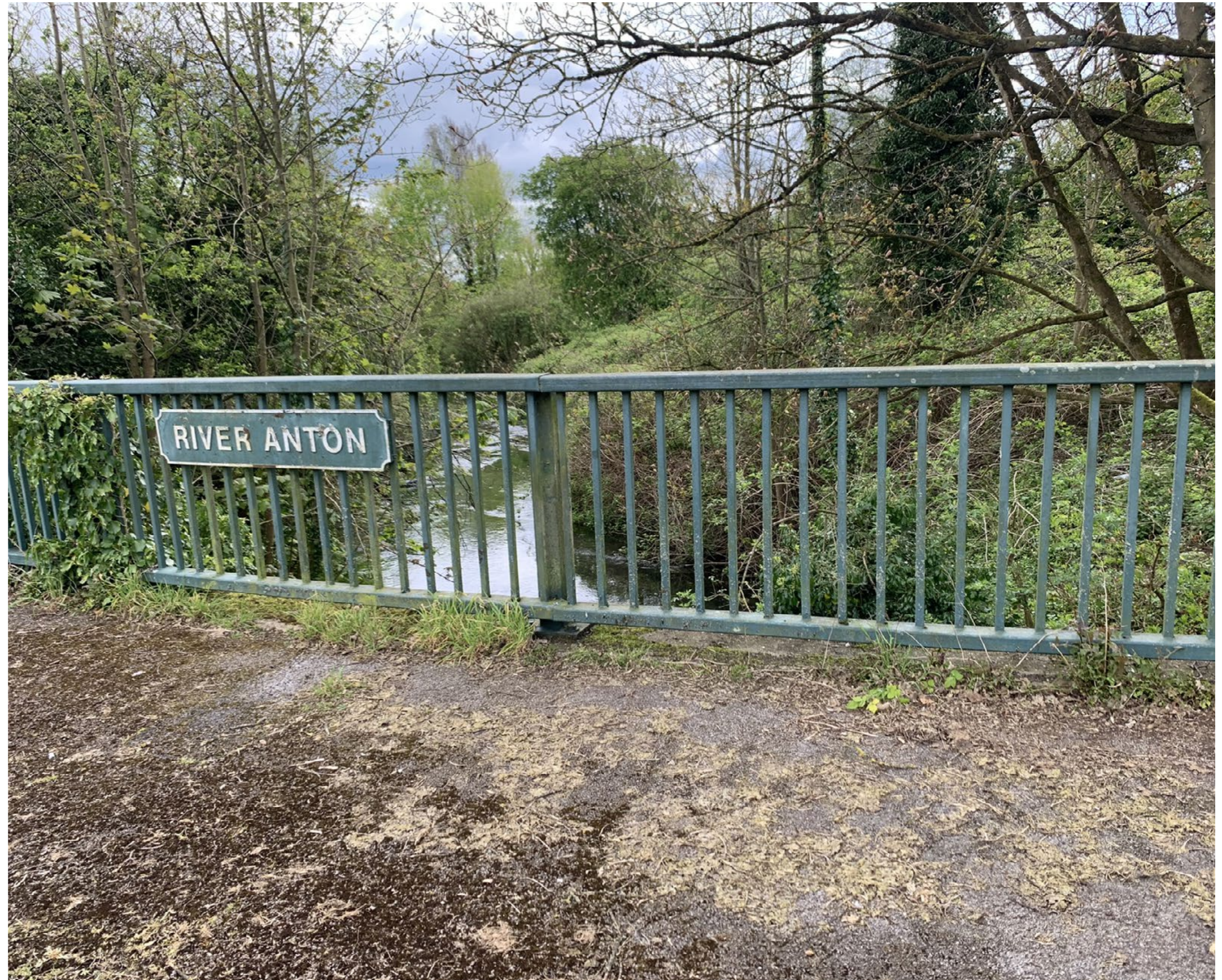
View looking South at the Western Avenue northern bridge
