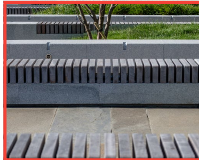
Timber seat on top of concrete wall
