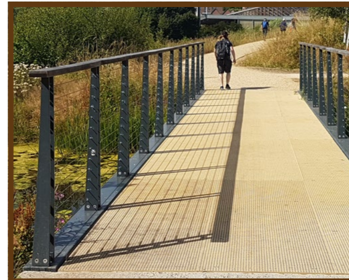
Metal balustrade - to promenades, for fall protection
