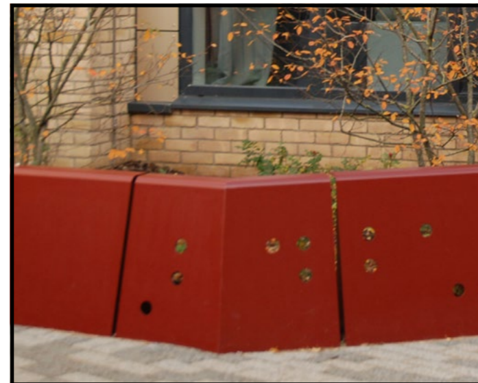
2) Metal wall - support for seating and play equipment
