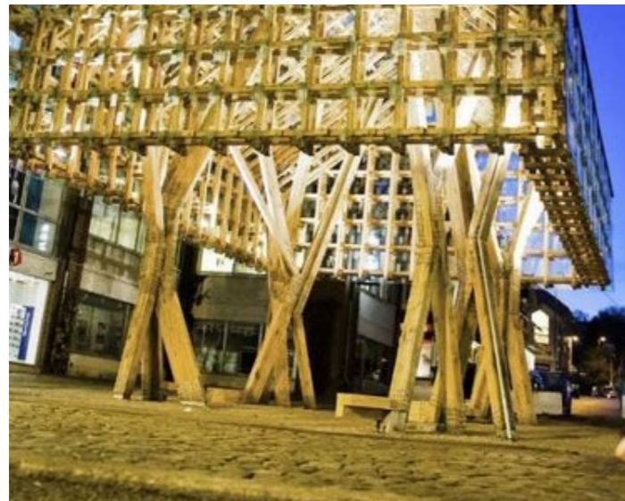
Simple structure with intricate columns (Photograph: Jonas Adolfsen)
