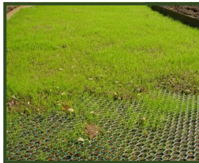
Reinforced lawn for maintenance vehicle access
