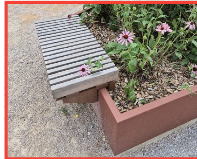
Timber seat on top of corten wall
