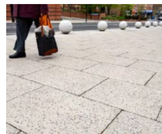
Footway / Enhanced precast concrete flag paving as typical street paving material outside of the Conservation Area.
