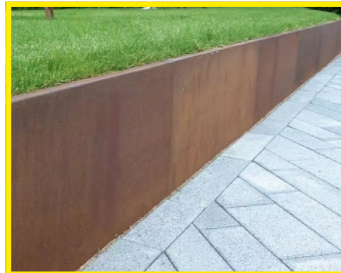
Corten sheet wall - to Southern entrance
