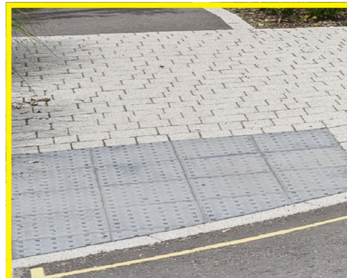
Tactile paving - Concrete pavers (to crossings and to cycle lane)
