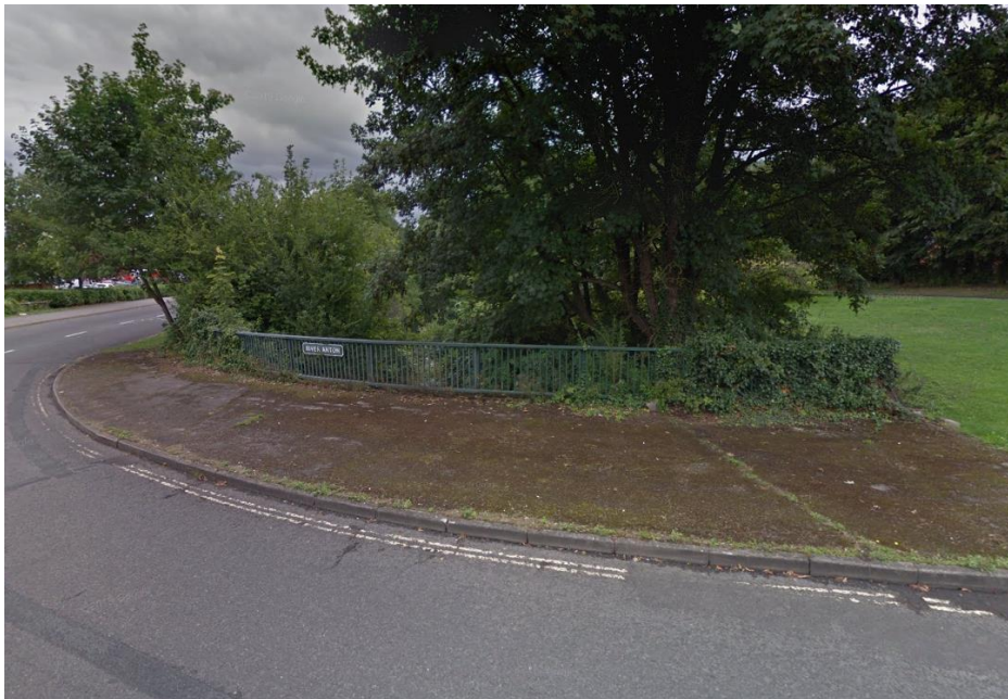
Figure 3 - River Anton Bridge Parapet (southern)
