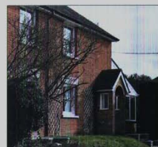
19th Century brick cottages, Winchester Street
