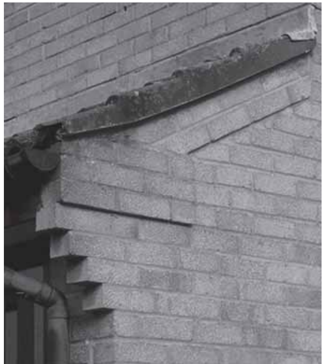
Brick detail in pale brick
