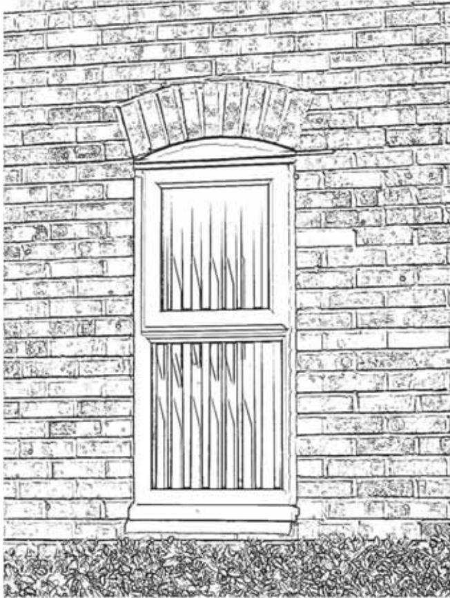
Window with fan bricks, Nursery Close
