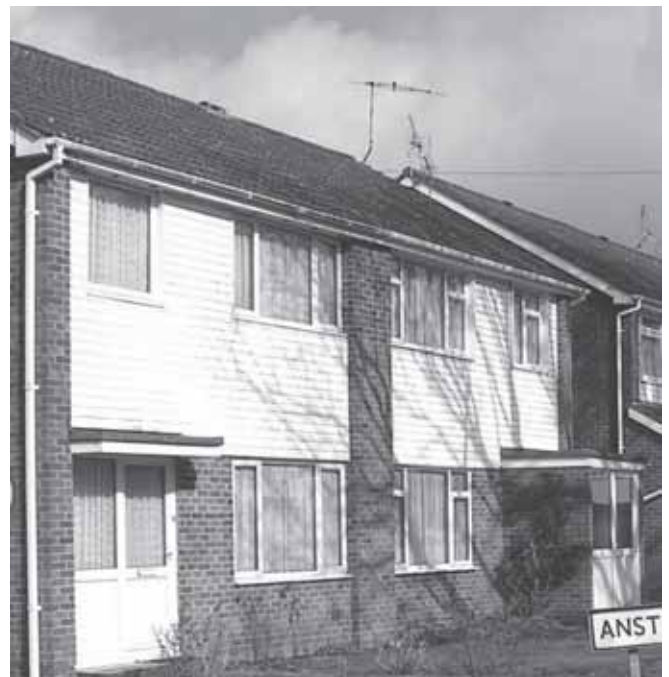
Shiplap and windows at the front of houses
