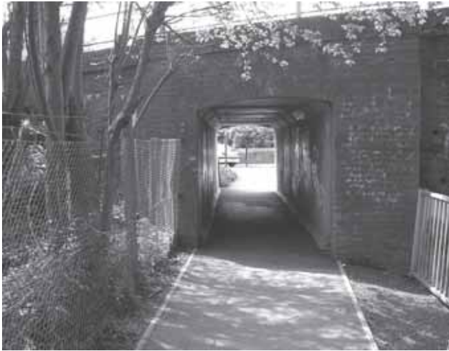
Railway tunnel beside Fishlake
