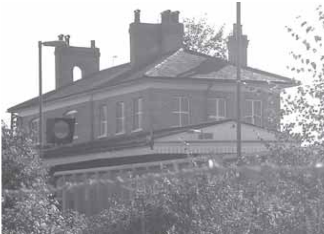
Railway station from the north
