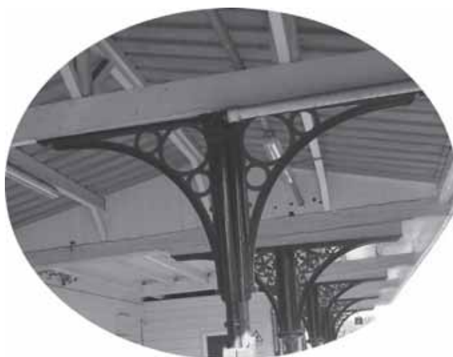
Roof supports in Romsey railway station
