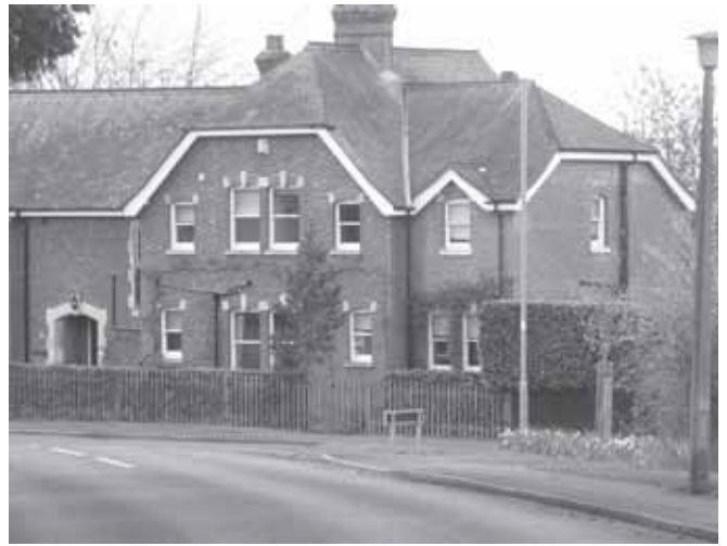
House in Cupernham Lane
