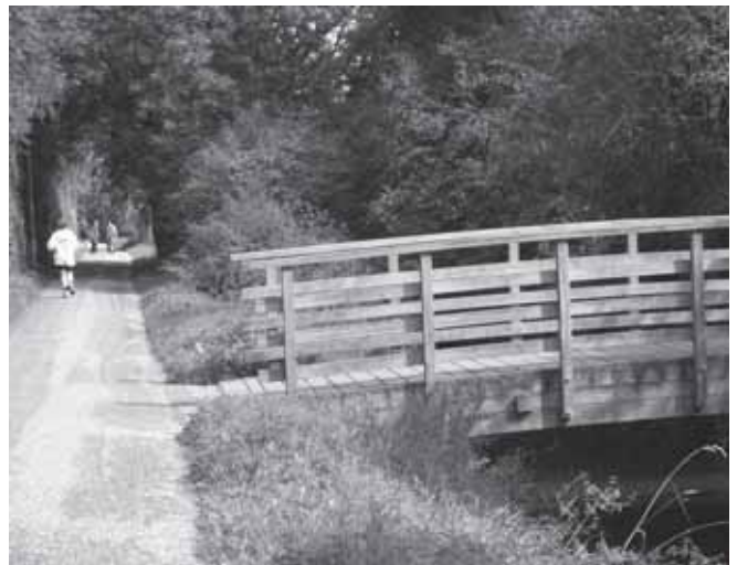
Mercer Way bridge over the Canal
