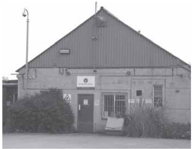
Canal Walk, Environment Agency depot
