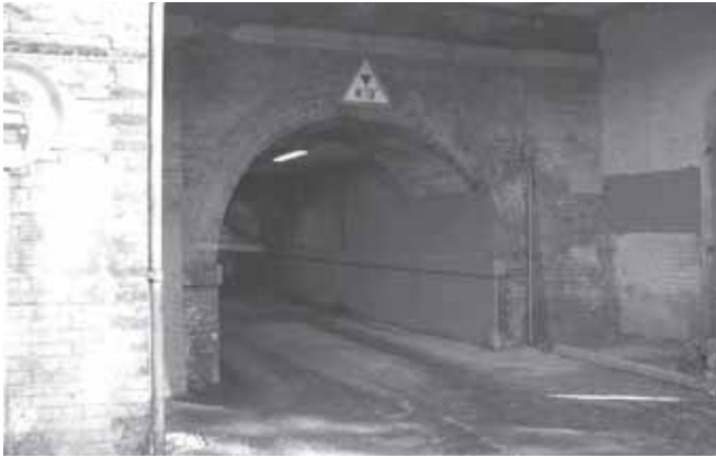
The approach to the railway tunnel
