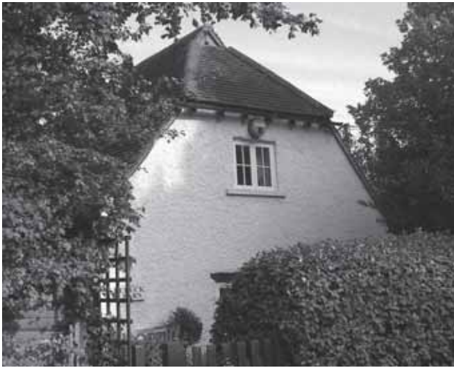
The Cruck Cottage in Cupernham Lane
