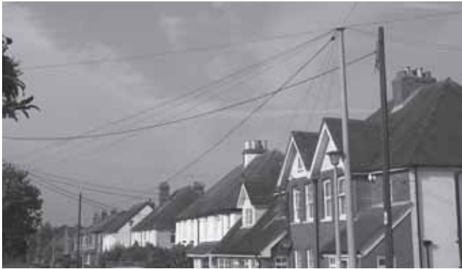
Cables in New Road
