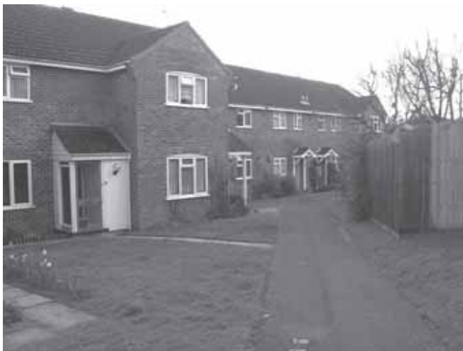
Brick facades in Dibben Walk
