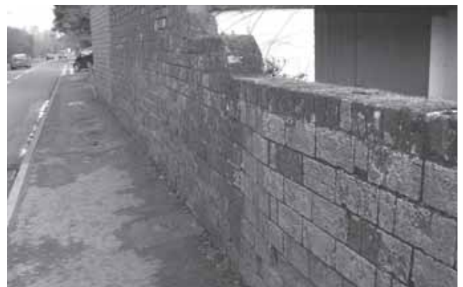
Brick wall in Braishfield Road
