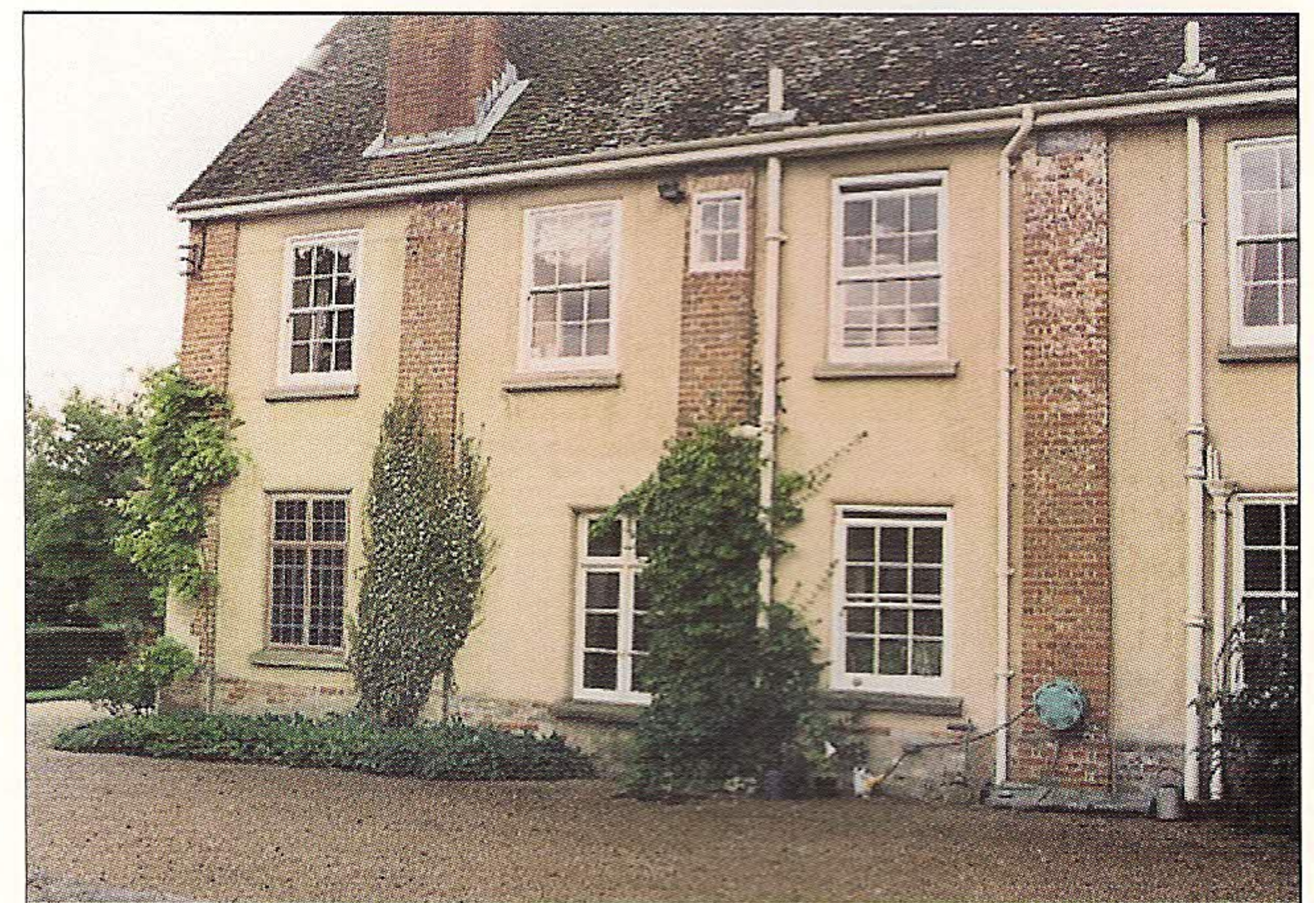
Carolean, Georgian and late Victorian windows on north wall: Penton Manor.
