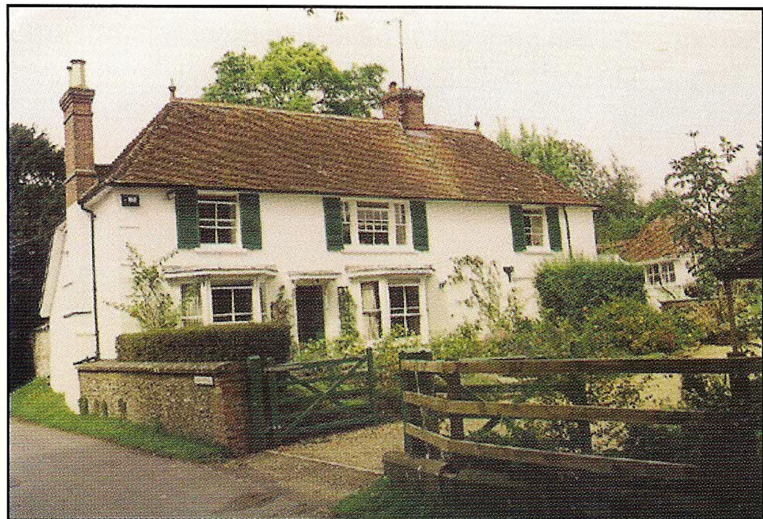
Cob and brick and flint walls: Folly Cottage.
