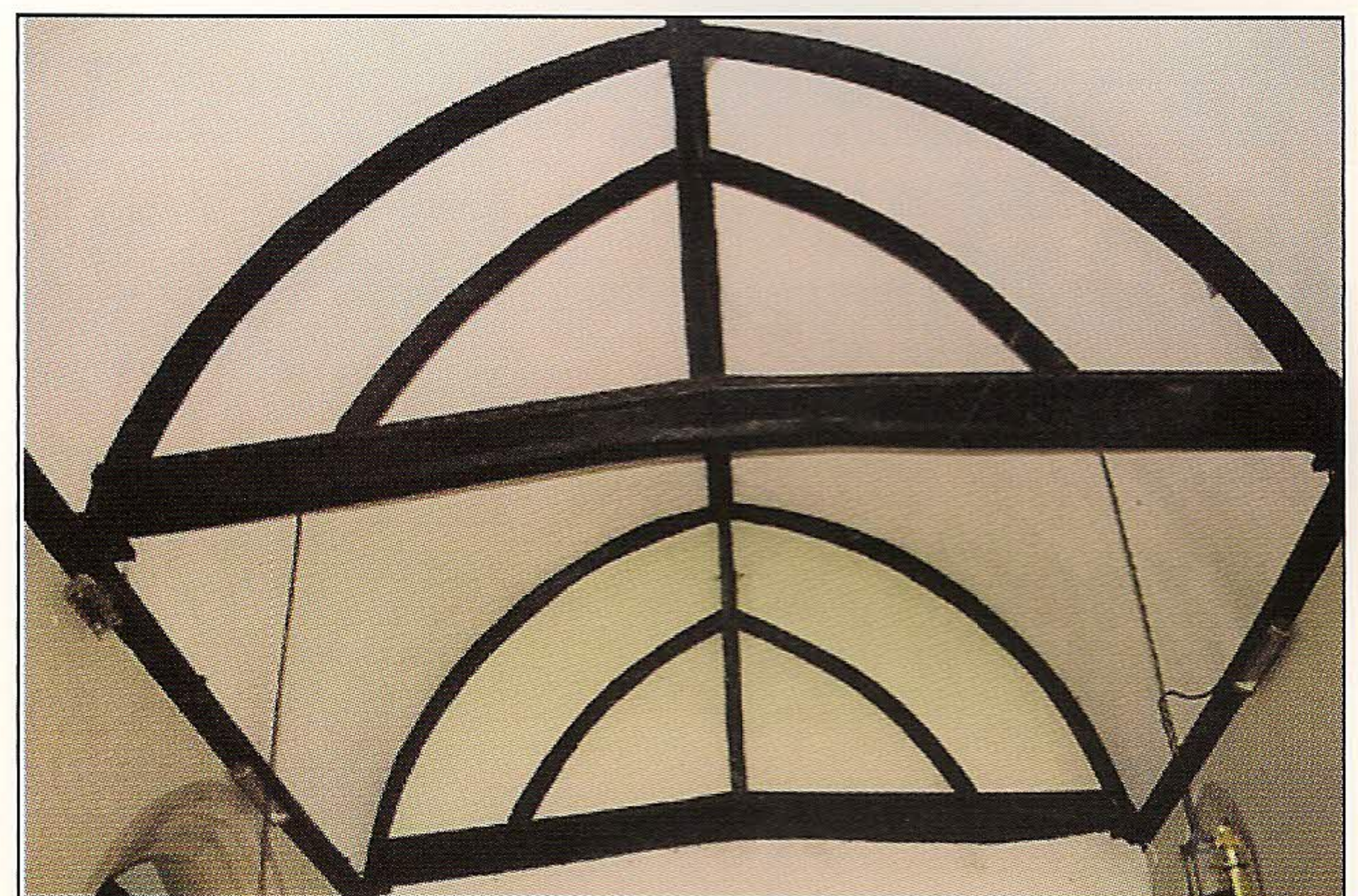
Interior of nave roof: Holy Trinity Church.
