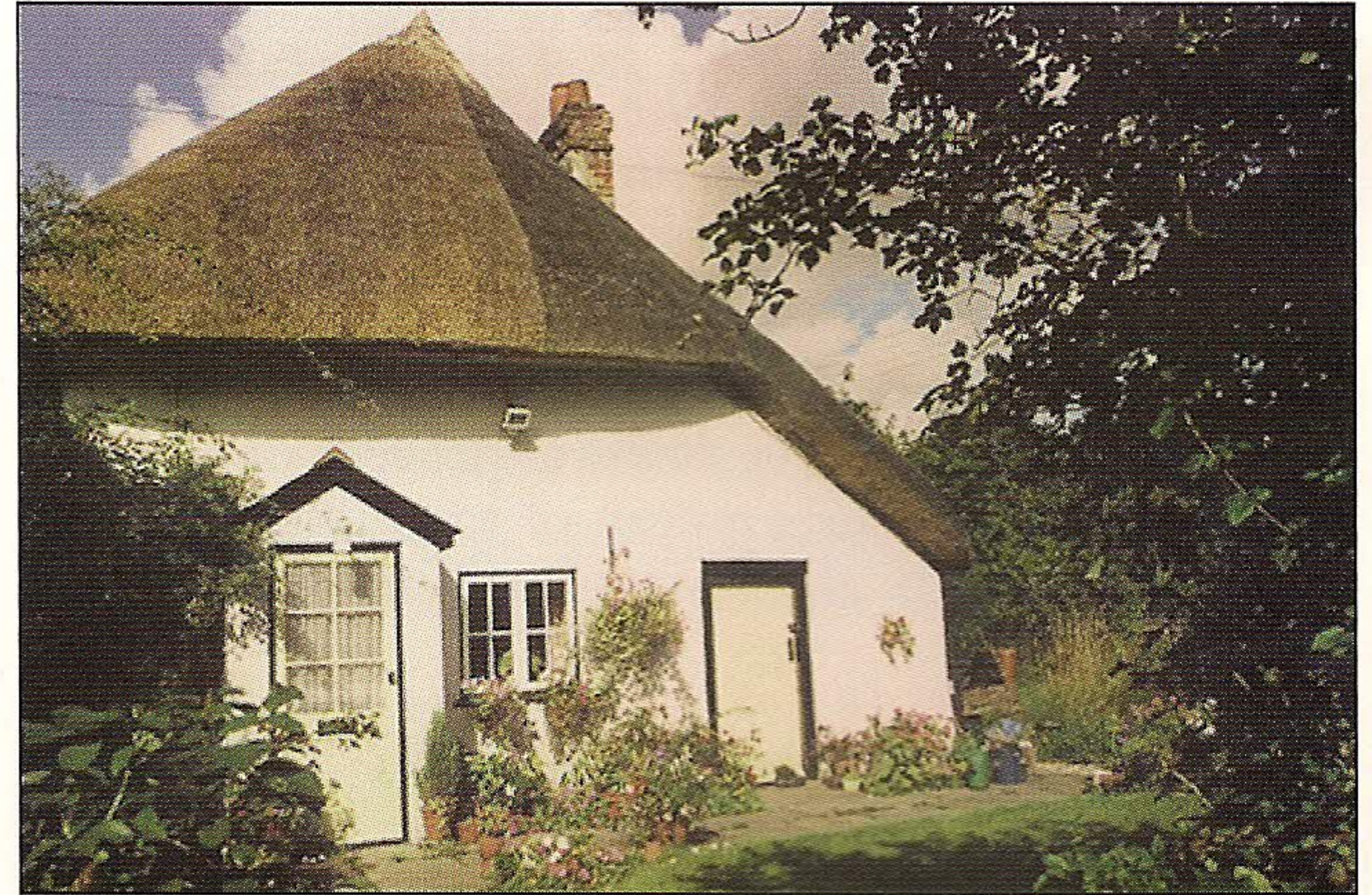
Casement windows and catslide roof: Sleepers Cottage.
