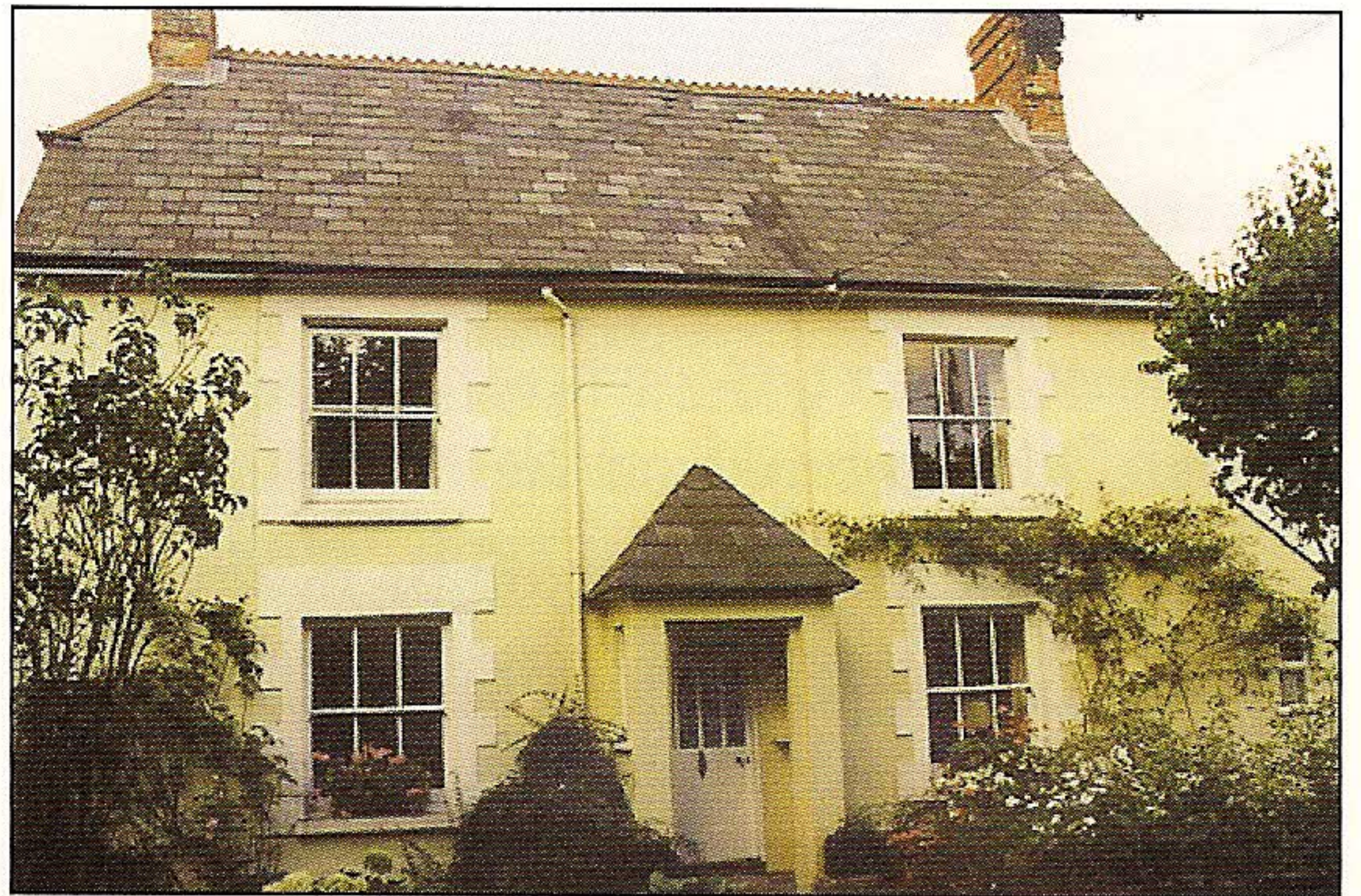
Slate roof and rendered cob walls: Walnut Cottage.
