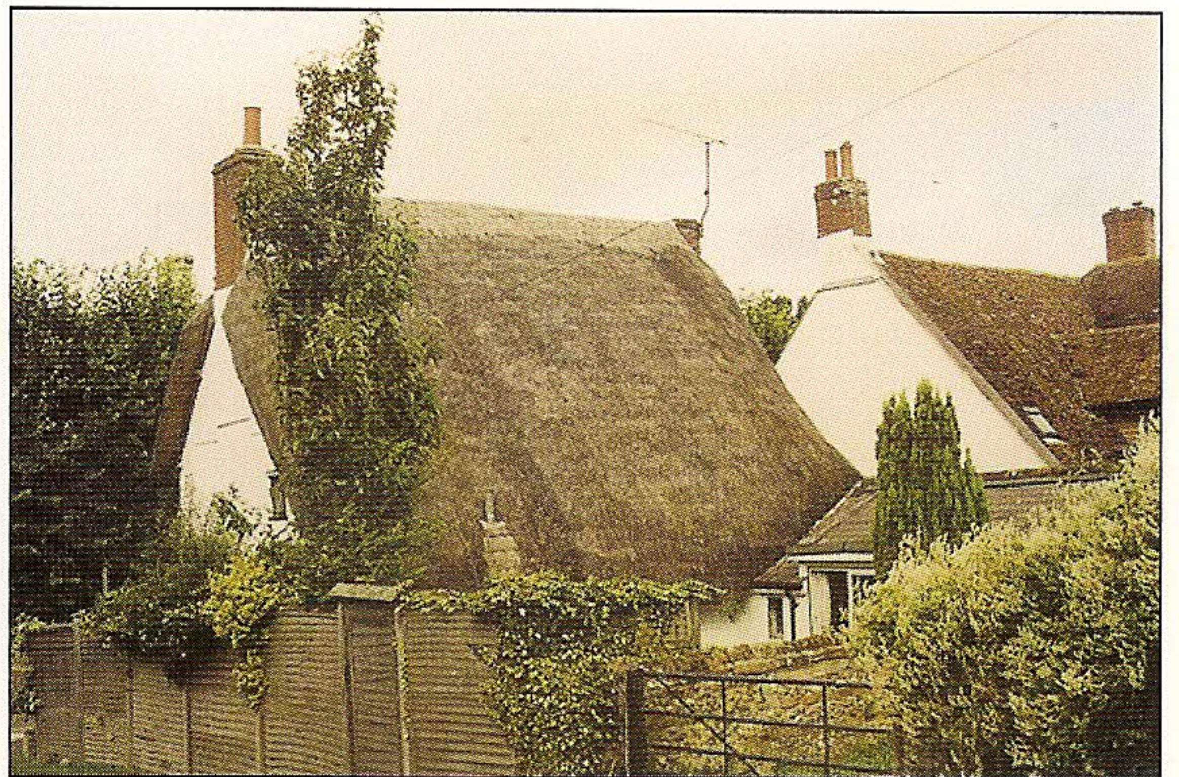
Thatch and catslide roof next door to tiles: Hillside Cottage and The Grange.
