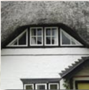
Triangular-shaped windows at eaves level
