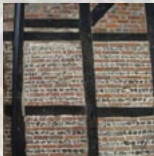
Timber-framing at Shilling Cottage
