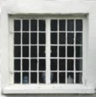
Small-paned metal window
