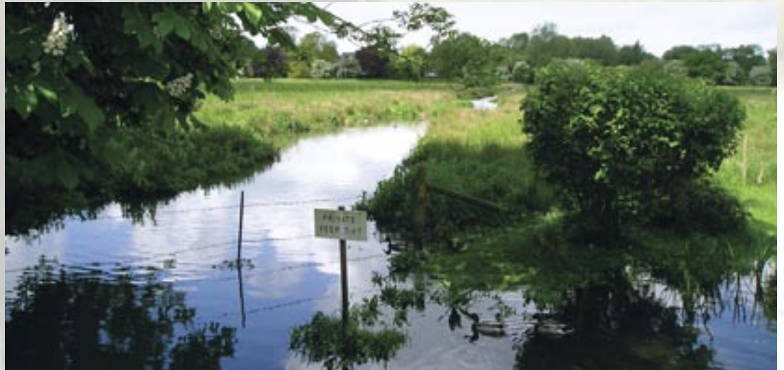
Sluice at Mill House
