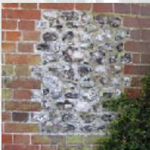
Brick and flint walling, Church Cottage, Amport
