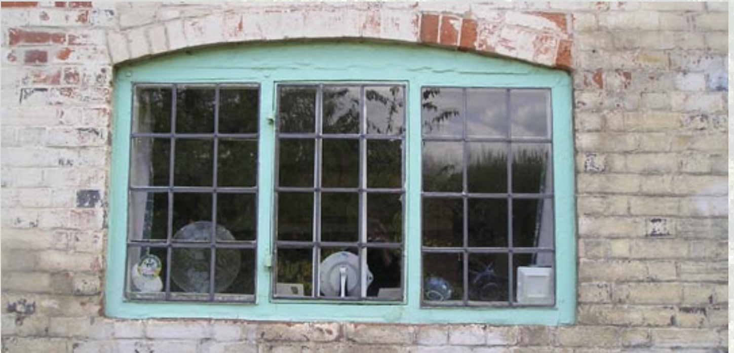
Metal Windows with leaded panels at Farm Cottage Monxton
