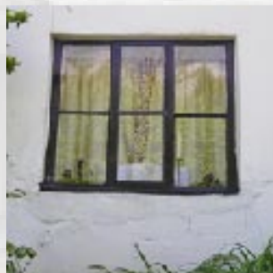
Hampshire Casement Window, Monxton
