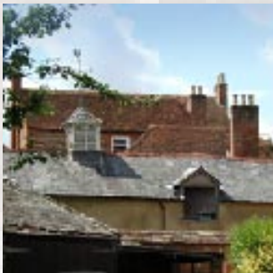
Clay tiles and slate roofing at Amport Firs
