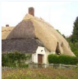
Thatching at April Cottage, Monxton
