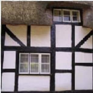
Timber framing, White Cottage, Amport
