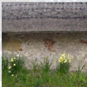
Cob walling, Old Farm House, Monxton
