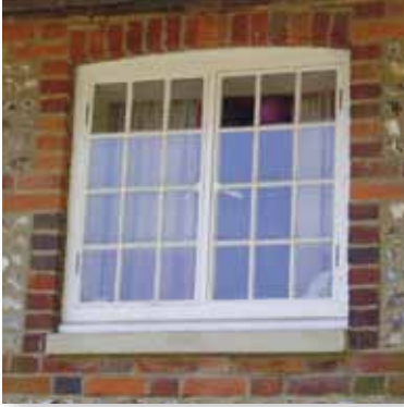
Metal casement window, Jesse Dewey Cottage
