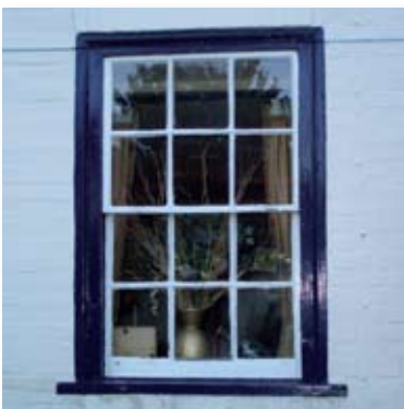
Sash window: Cricketers Inn
