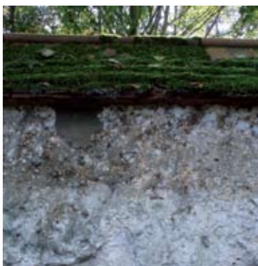
Cob wall: Stableyard at Longparish House
