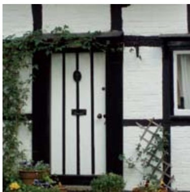
Timber framing: Inglenook Cottage Forton
