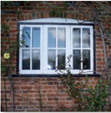
Casement window: Rose Cottage
