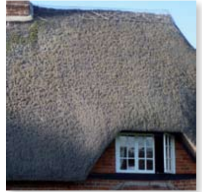
Thatched roof: The Old Curacy
