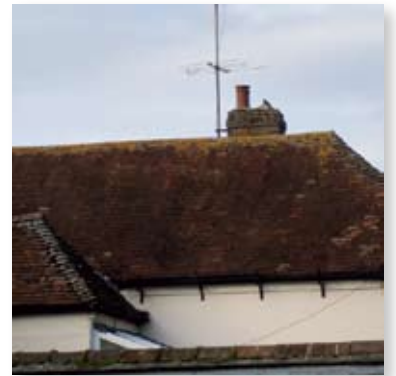
Clay tile roof, The Grange
