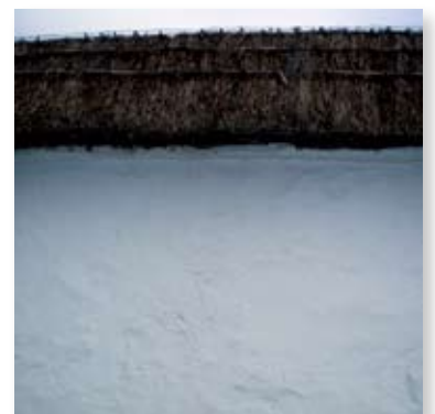
Cob wall, The Cottage
