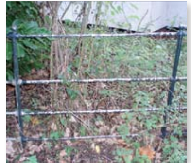
Estate fencing, Penton Lodge
