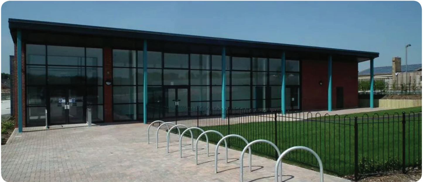
Above: The new Picket Twenty Community Centre on Picket Twenty Way
