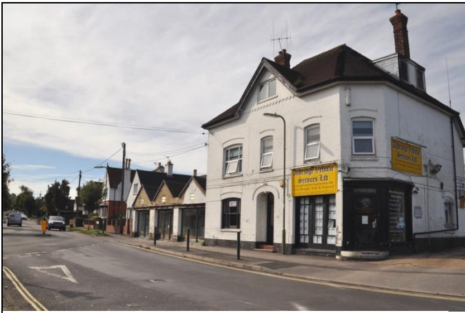
Figure 1B -13 View south west towards the two and a half storey white painted brick corner building
