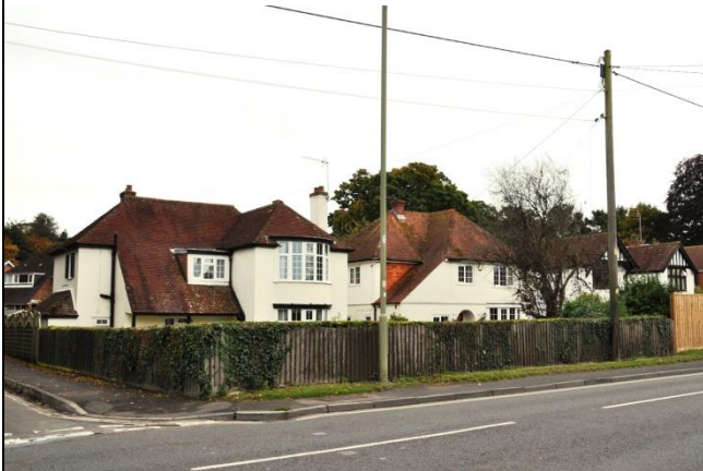
Figure 2C -15 Looking south towards the distinctive group of white painted rendered houses to the south of the junction of Winchester Road and Winchester gardens
