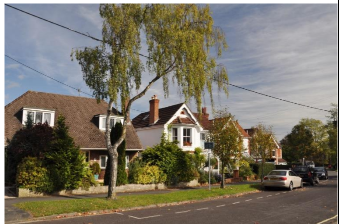
Figure 2C-10 Looking east. Note to the right of the view the pre-war houses on the north side of the street. These have gabled fronts, bay windows, ornate bargeboards. Most also have stonework/brickwork quins. The sequence starts with number 10, the rendered white painted house
